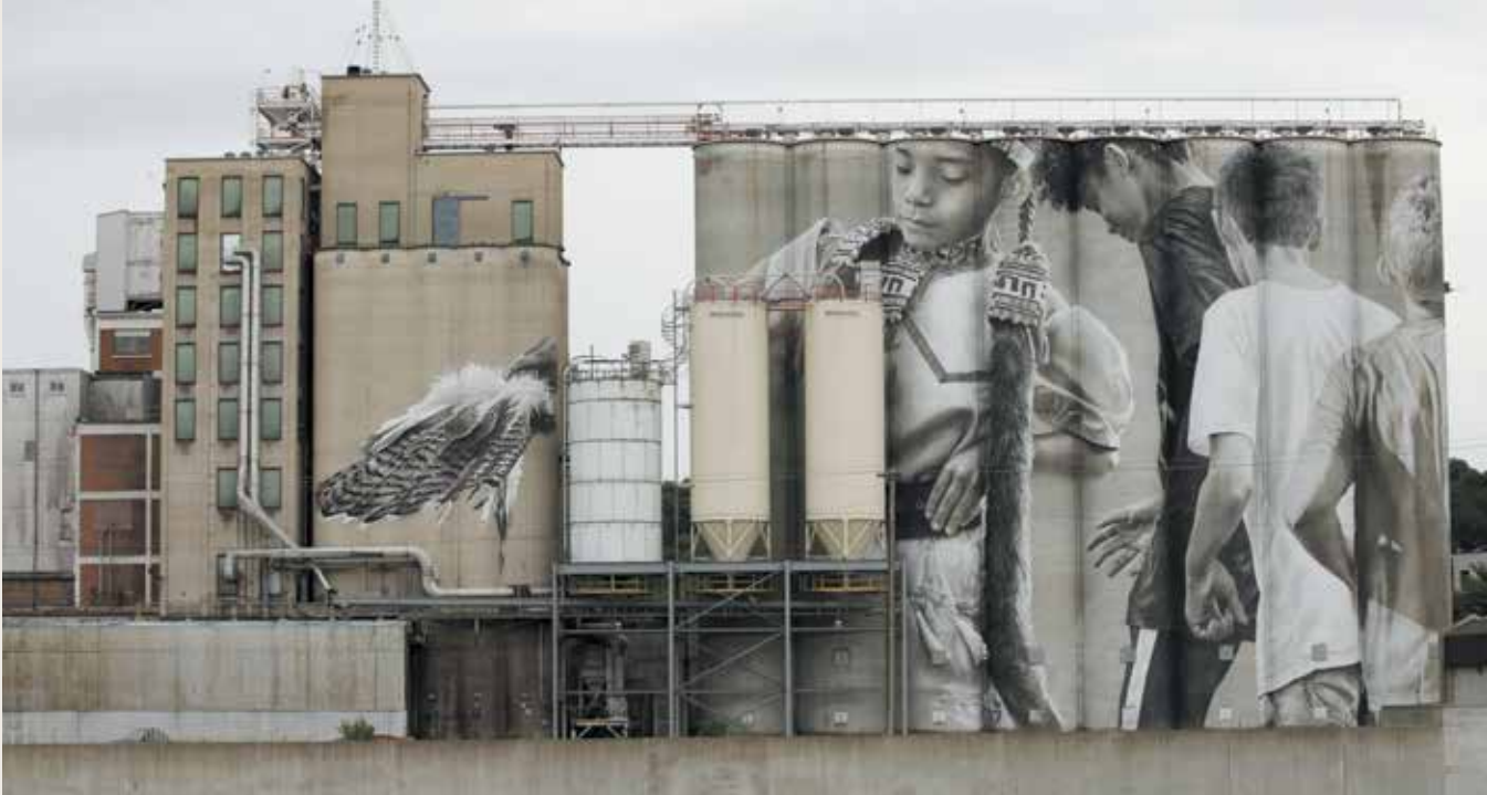
VIEW OF SILOS FROM NORTH MANKATO
